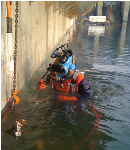
Getting His Feet Wet. A diver prepares to do some welding at The Dalles Lock and Dam on the Columbia River.
